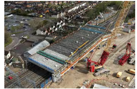
Bletchley Flyover, May 2021 courtesy of NR Air Ops
